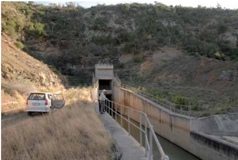
Figure 22. The exit point of the tunnel which carries water via the Hermanuskraal Weir, Great Fish River, to the Glen Melville Dam (photo: Jim Cambray; 31 July 2008)
