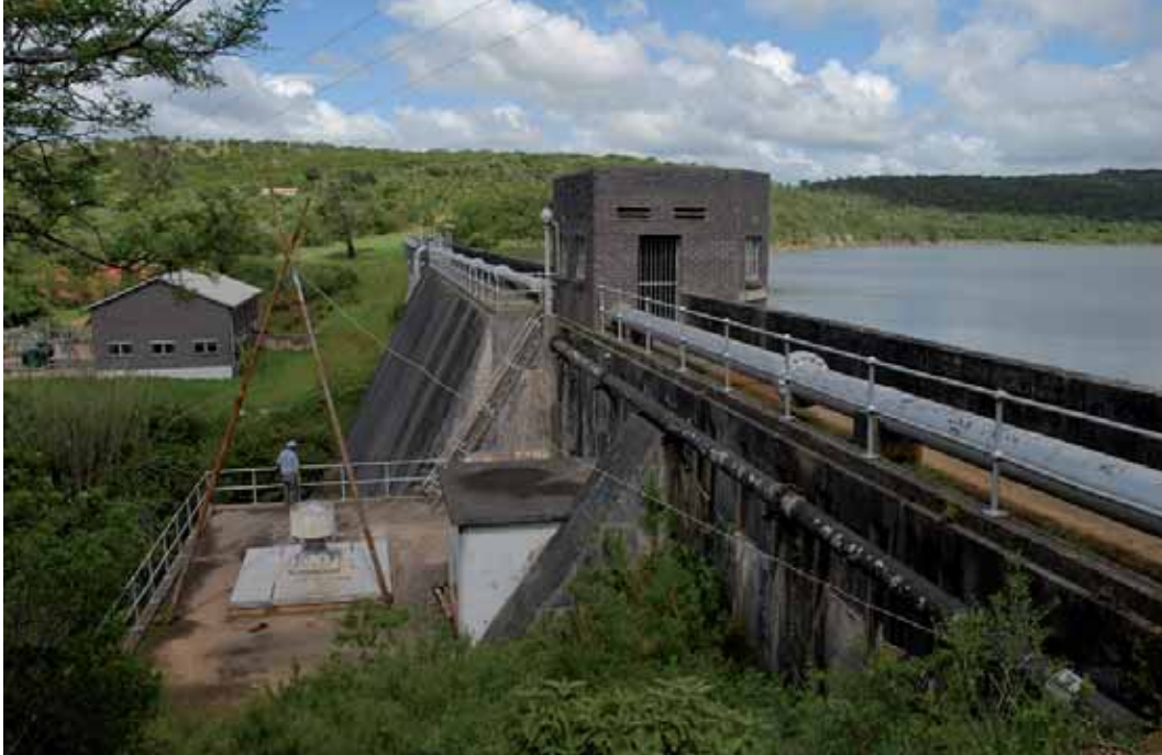
Figure 14. Howison’s Poort dam wall with the old pumping station in the foreground and the new pumping station in the left background (photo: Jim Cambray; 18 January 2008)
