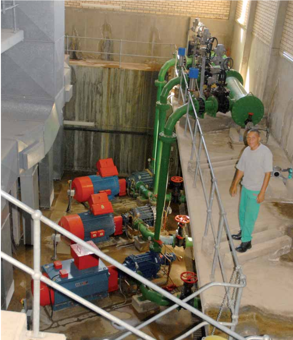
Figure 24. Mr Phillip Nobomvu points towards the heart of the Jan Kleynhans water treatment plant: the three large pumps that keep water circulating at 125 litres per second. If any one of these fails then the main pump, closest to Mr Nobomvu, will turn on (photo credit: Jim Cambray; 31 January 2008)
