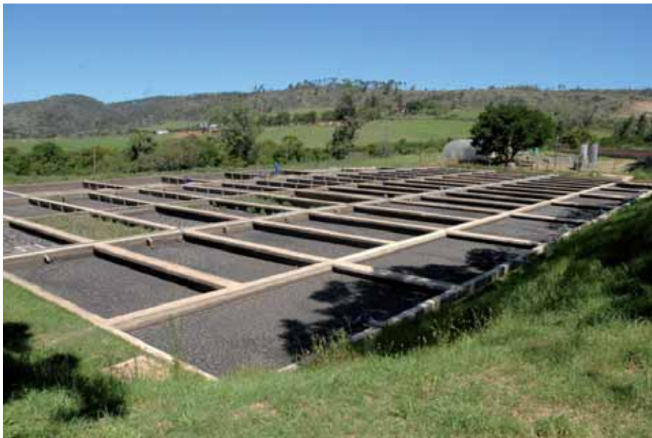
Figure 27. The Belmont Valley sewage plant (photo: Jim Cambray; 30 January 2008)
