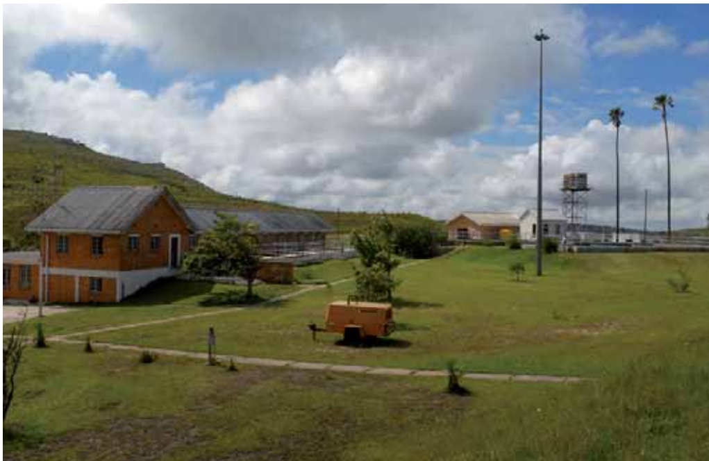
Figure 17. Waainek filtration plant: on the right (below palms) are the settling ponds; the brick building at the back and the white building are used for storing alum and lime store, respectively; the building on at the left front houses the filtration plant, where chlorine is added (photo: Jim Cambray; 18 January 2008)
