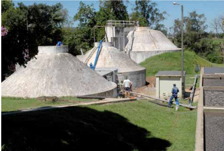
Figure 26. Three digesters at the Belmont Valley sewage plant (photo credit: Jim Cambray; 30 January 2008)
