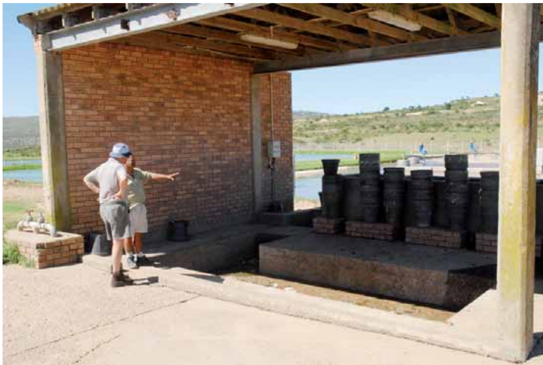
Figure 25. The superintendent of the Mayfield sewage works discusses the termination of the bucket system with the author. Mr Wessels noted on 30 January 2008 that only 200 households were still serviced by this system (photo: Jim Cambray; 30 January 2008)
