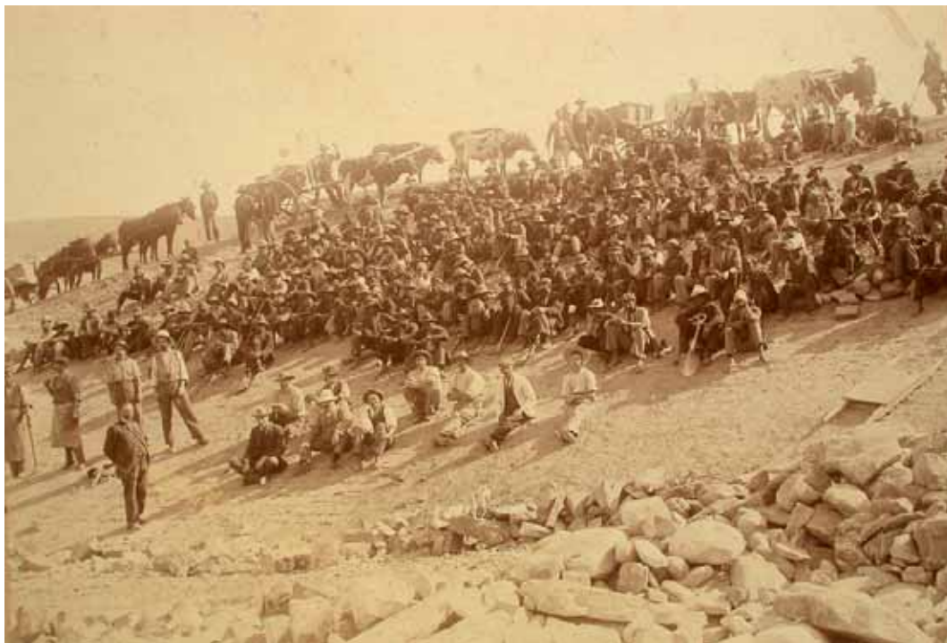
Figure 11. Undated photograph taken by the old firm of Hepburn & Jeans (circa 1897) showing progress in the construction of either Milner, or Jameson, Dam. There are at least 120 workers at rest on the bank. Note the ox- or mule- drawn scotch-carts, which could be tipped to release their payloads. In the foreground stands an imposing figure, perhaps the engineer (Albany Museum Archives: SM Pic. 5801)
