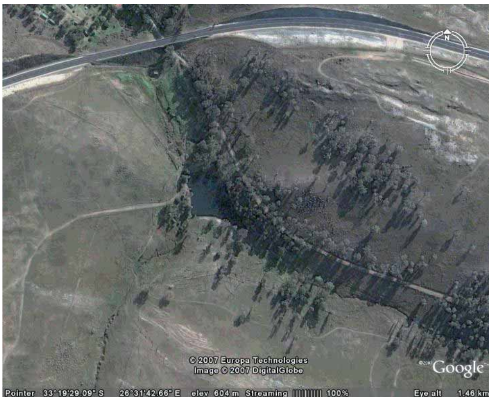
Figure 4. Grey Dam (downloaded from Google Earth )
