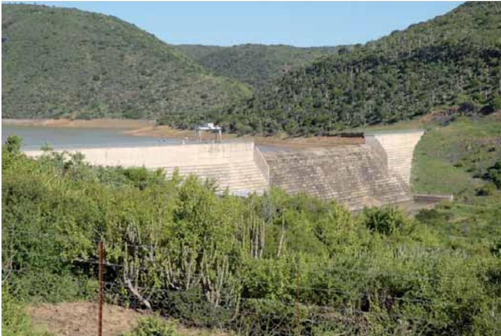
Figure 19. Glen Melville dam wall (photo: Jim Cambray; 31 July 2008)
