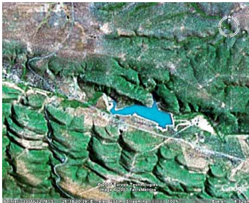
Figure 18. Glen Melville Dam with filtration and pumping station east of the dam wall (downloaded from Google Earth; 18 September 2007)
