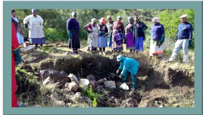
Community members being taught by a peer on how to construct a stone pack to arrest headward erosion
