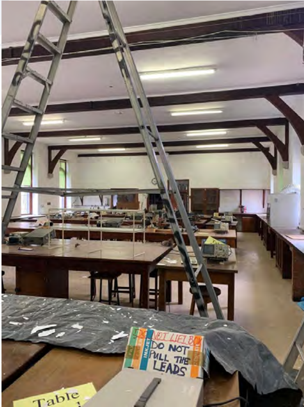
Laboratory space at Physics being renovated to receive the BRG
