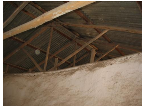
3e. Inside view of corrugated iron roof.
