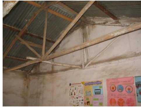
3e. Inside view of corrugated iron roof.
