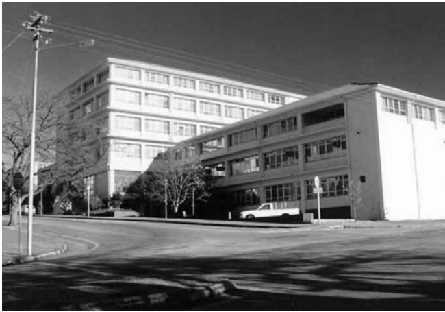
Figure 23. The Zoology & Entomology building in 1993 after the removal of the shutters and addition of floors. Photograph by A.N. Hodgson.
