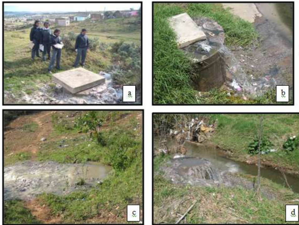
Figure 16 (a) Wastewater leak near a school in Grahamstown East (Courtesy of the KCC) (b) Sewerage running into the Bloukrans stream (Courtesy of the KCC) (c ) Leak in Raglan road from a wastewater manhole (Courtesy of the KCC) d) Sewerage overflow off Beaufort Street (own image)
