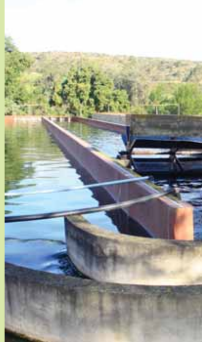
High Rate Algae Oxidation Pond (Raceway) - a component of the Algae Integrated Pond System used for the treatment of domestic waste water
