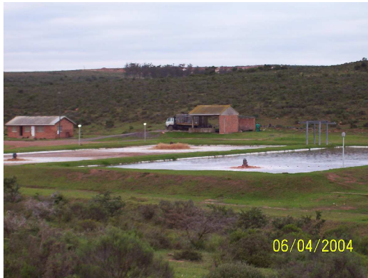
Figure 13. Mayfield STW showing ponds with aerators, sludge, buckets and inlet
