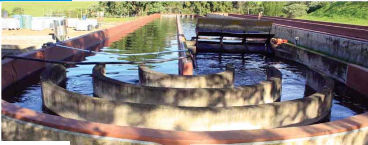
High Rate Algae Oxidation Pond (Raceway) - a component of the Algae Integrated Pond System used for the treatment of domestic waste water.
