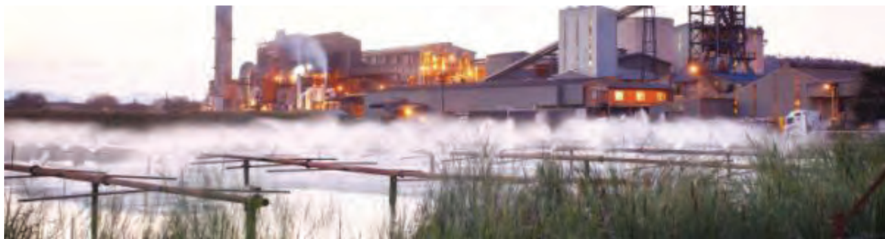
A view of TSB Malelane Sugar Mill, Nelspruit, spray dams to cool water used in phases of sugar manufacturing before it is released back into the resource (at Stingspruit channel into the Crocodile River).
