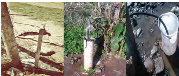
Leakages and broken taps are common in Nomathamsanqa (picture 1) and Aquapark (picture 2 and 3)
