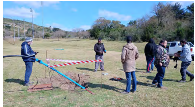
Plate 1: The IWR team, Djim Diongue, Jacobus van Jaarsveld, Phatsimo Ramatsabana and others preparing to conduct borehole pump tests to determine sustainable pumping rates for Rhodes.
