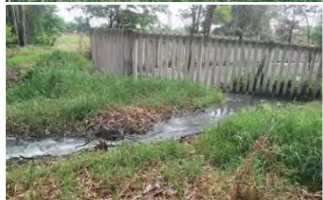
Overflow of raw sewage caused by failure of Pumping Station 8 in Vereeniging (Photograph by Noleen Tavengwa, 8 October 2021)
