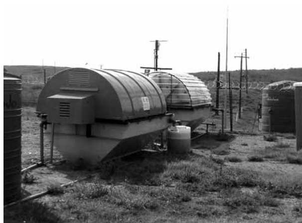
First and second contacting rotators in series for mine water treatment at Middleburg, Mpumalanga - TIA project in collaboration with UBA Biologix.
