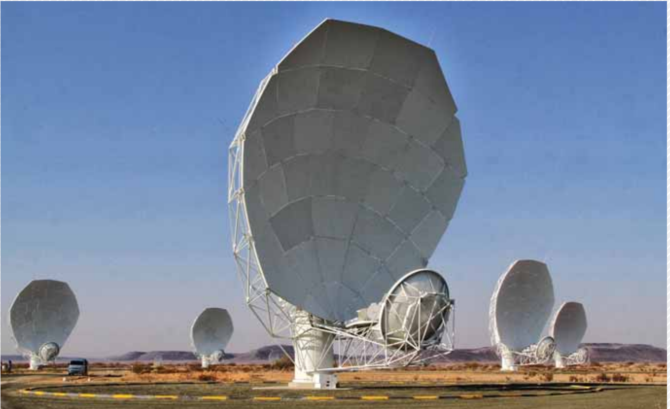
The MeerKAT dishes, made up of discrete panels, are carefully engineered to offer a smooth surface Credit: Chris Marais
