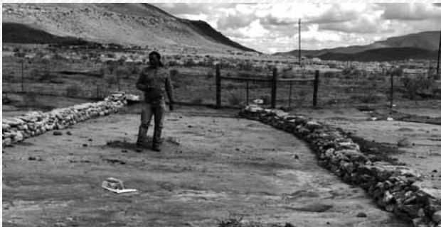
Simple rehabilitation methods using stone lines in Machubeni, Eastern Cape Credit: Department of Environmental Science
