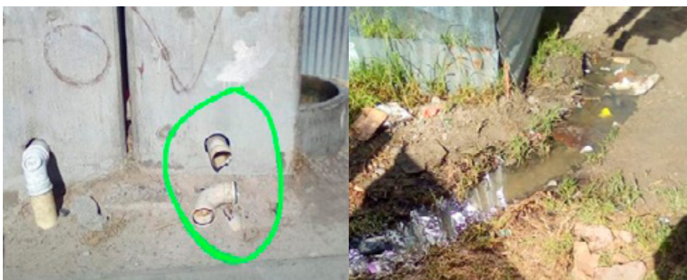
Left: Mfuleni – broken toilet pipes Right: Mfuleni – sewage in the street
