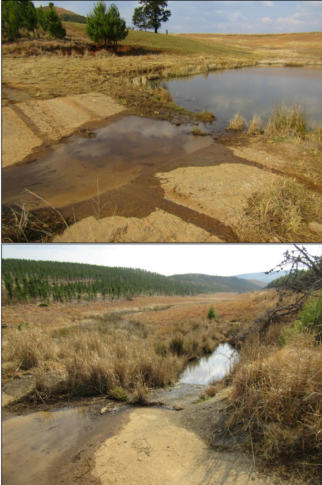
Figure 4: A well maintained and vegetated spillway
