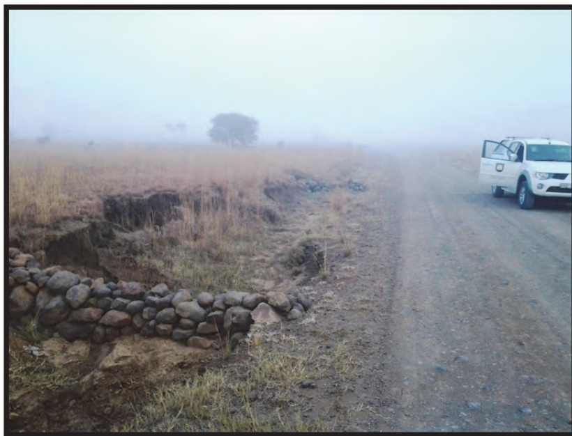
Figure 2.22: Efforts to stop erosion along the road (Located at Photo 7 in Figure 2.2).
